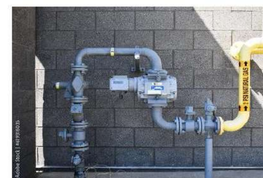
Dresser Natural gas meter with low psi piping
