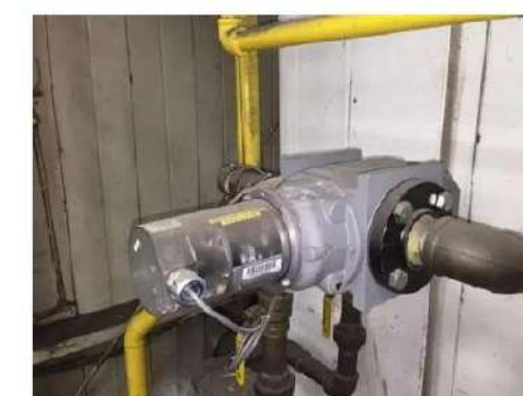
Sub-Metering Natural Gas in a Factory Control Environment
